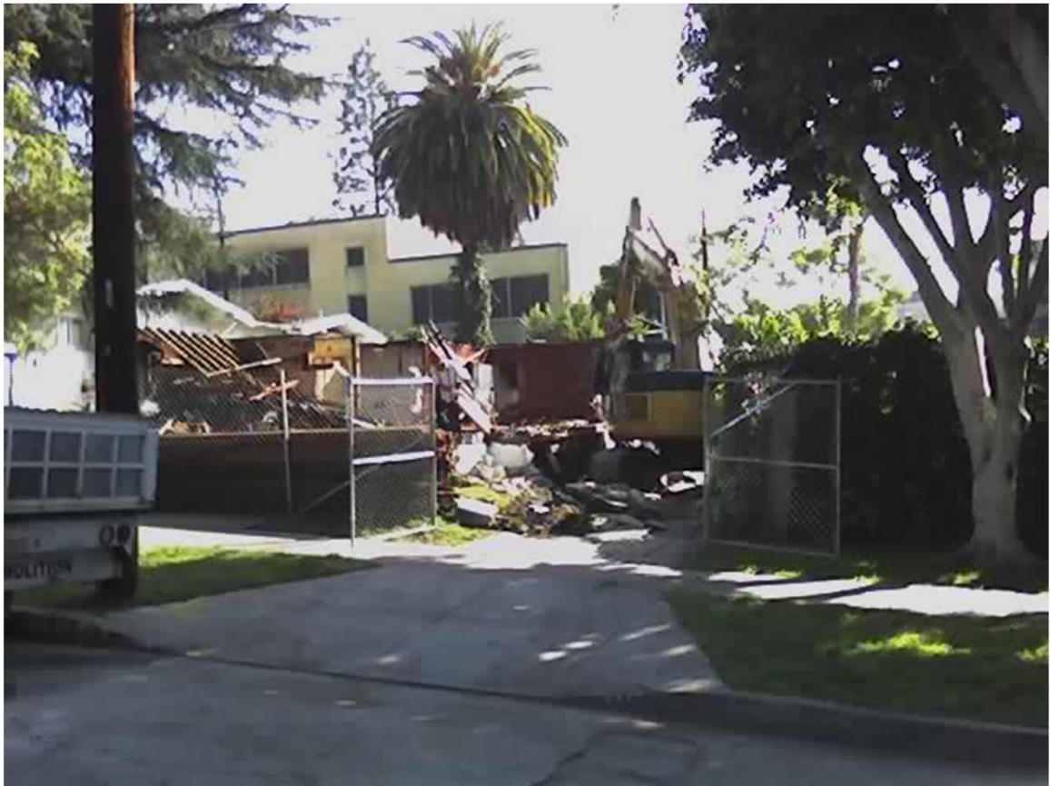
1912 St Andrews- after demolition
